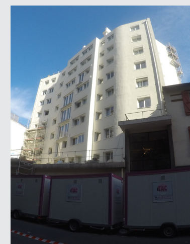
FAÇADE APRES RENOVATION
